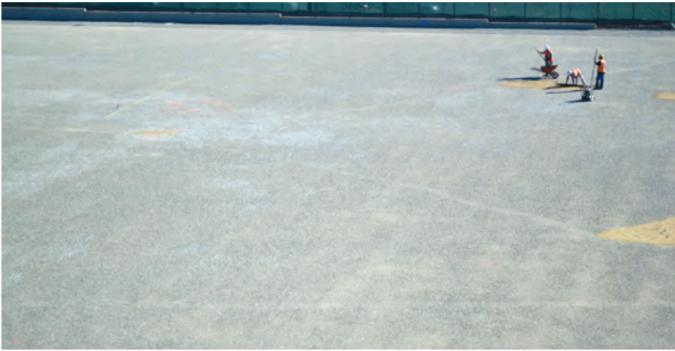
OHNO construction workers make sure that gravel is consistently flat and level before the grass can be placed on the field.
