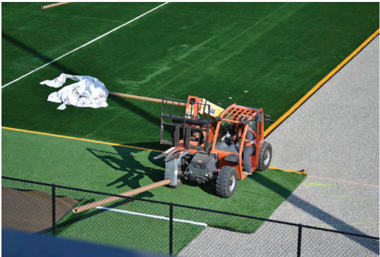
OHNO construction workers and FieldTurf Co. install the polyurethane grass and insert grass sections with colored lines that are sport specific.
