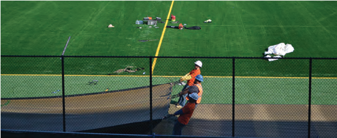
FieldTurf construction workers drag the polyurethane grass across the side of the main field.
